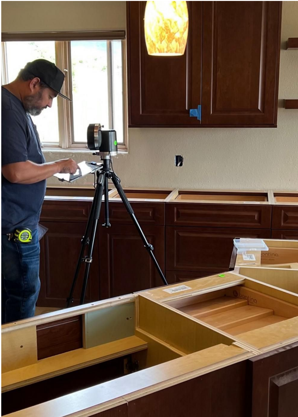
Digital templating equipment is a reliable method for fabricators to achieve speed, accuracy and complex work. Photo courtesy of Laser Products Industries
